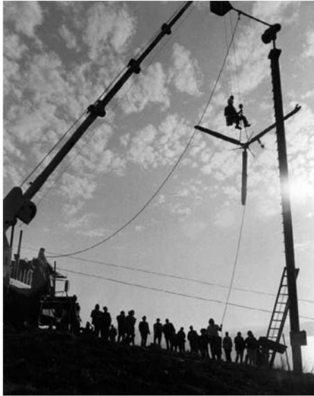
Above, 6 kW wind generator erected by Interactive Resources in Point Richmond was first in California to cogenerate. It was extensively instrumented and monitored by PG&E. Below, home using solar water and space heating featured on cover of Sunset Magazine
