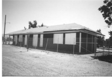
CENTERVILLE DEPOT IN 1997 (PRE-RESTORATION)
