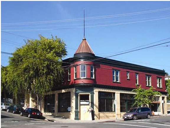
201 West Richmond Avenue, owned and rehabilitated by Mark Howe
