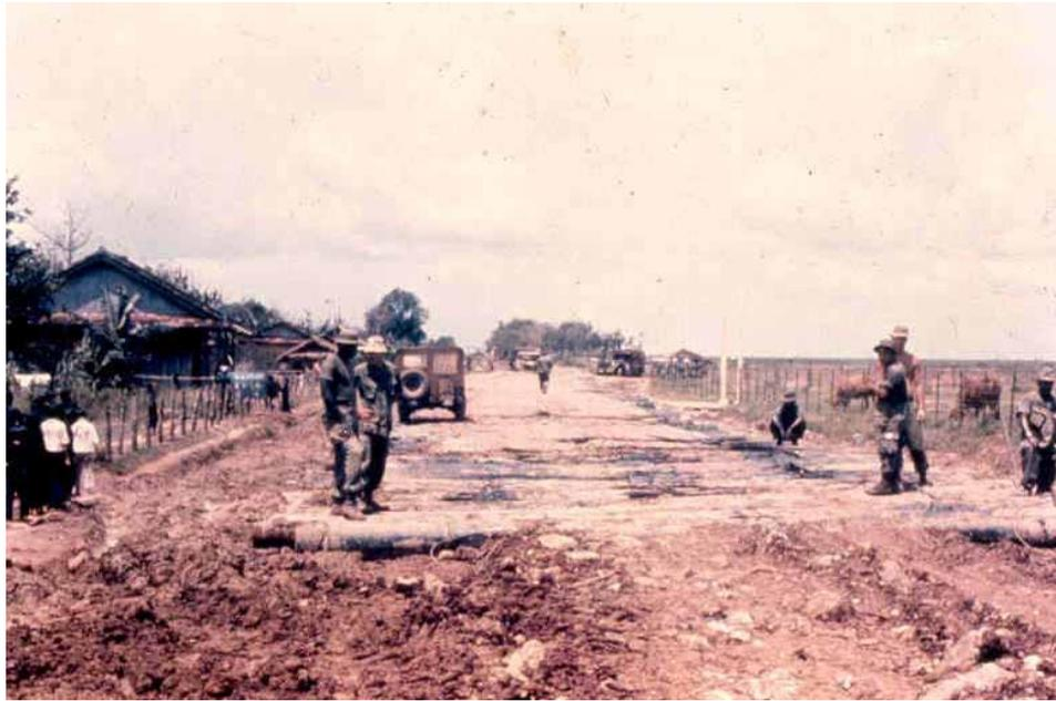
*Figure 78 - Military Service Road (MSR) Zinc – placing corduroy road, 34<sup>th</sup> Engineer Battalion, September 1969. A “corduroy road” is an ancient technique of using tree trunks lined up side by side to provide support on muddy soil.*
