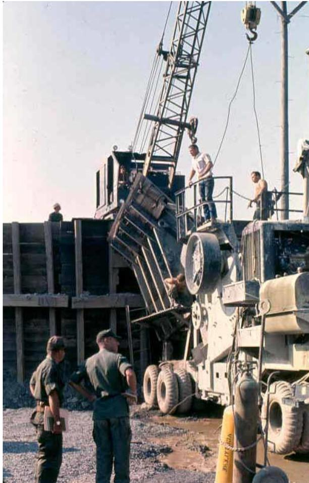
*Figure 73 - Asphalt plant at Phu Hoi operated by 34<sup>th</sup> Engineer Battalion, December 4, 1969*
