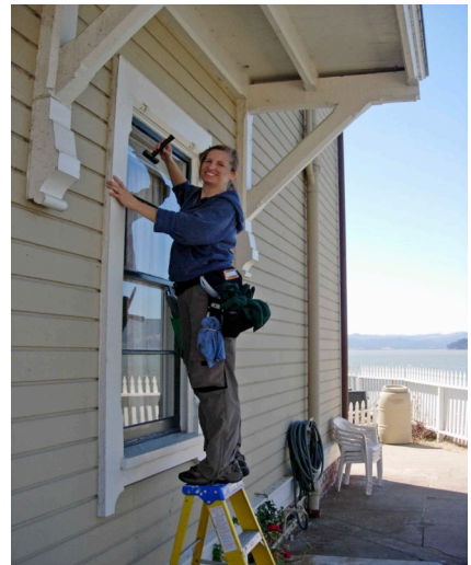
A 4 inch razor blade scraper gets the salt off the windows
