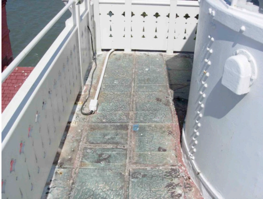
Original copper deck covering
